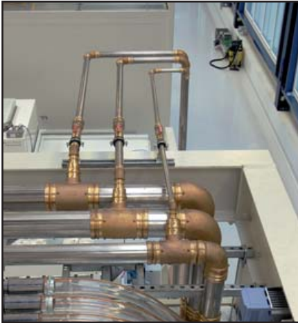
Optipress, the easy-to-assemble and economical sanitary installation system, is based on the most modern press-fit technology
