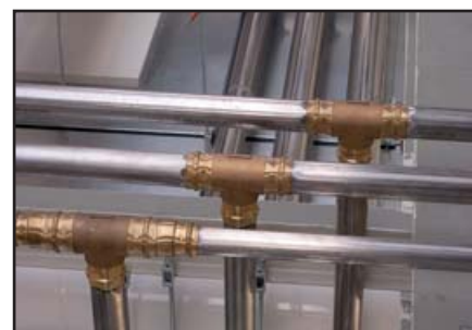
Optipress pipes of stainless steel with fittings and fixtures of gunmetal
