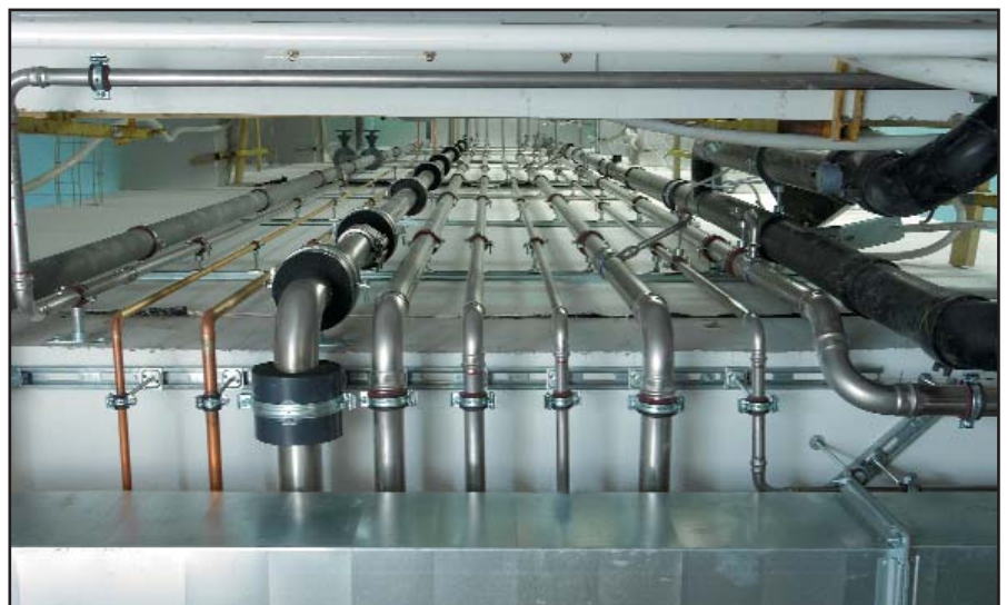
Vertical service shaft
