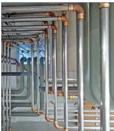
Optipress in the riser zones of the main distributors TZ 12
