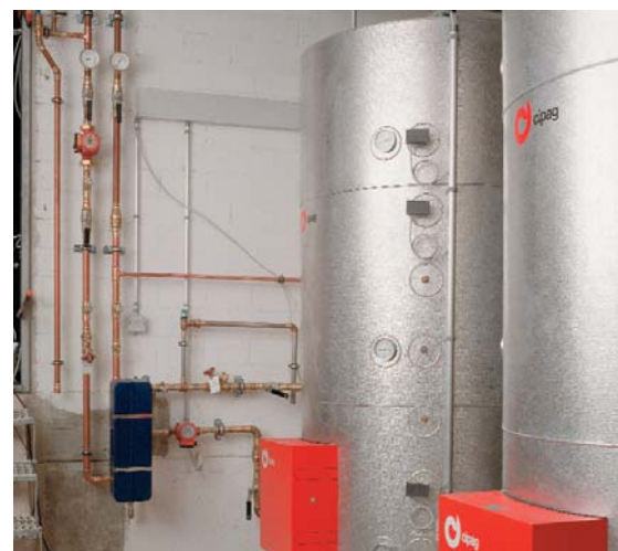
The solar installation's twin hot water storage tanks, with incoming and outgoing pipes using the Cupress installation system.
