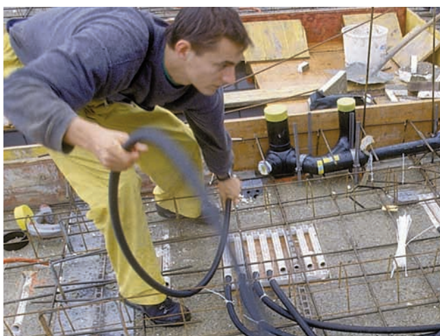
Optiflex-Einlegetechnik inklusive // Technique d'insertion Optiflex incluse // Posa in getto Optiflex inclusa
