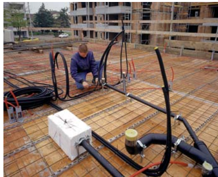
Laying Optiflex pipes to the individual apartments.
