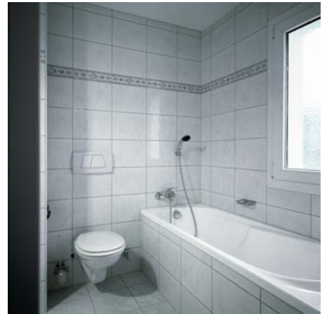
The flexible Optivis masking-wall system was used for all of the bathrooms.
