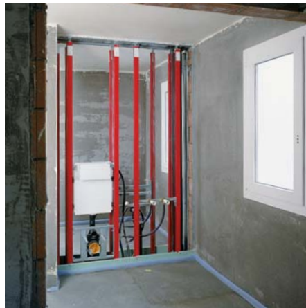
The flexible Optivis masking-wall system was used for all of the bathrooms.
