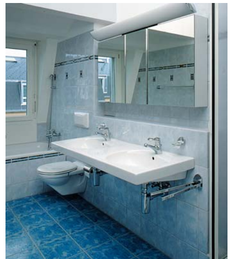
Bathroom installed using Optivis.
