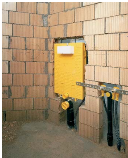
Optibloc "brick" modules were used in the small bathrooms.
