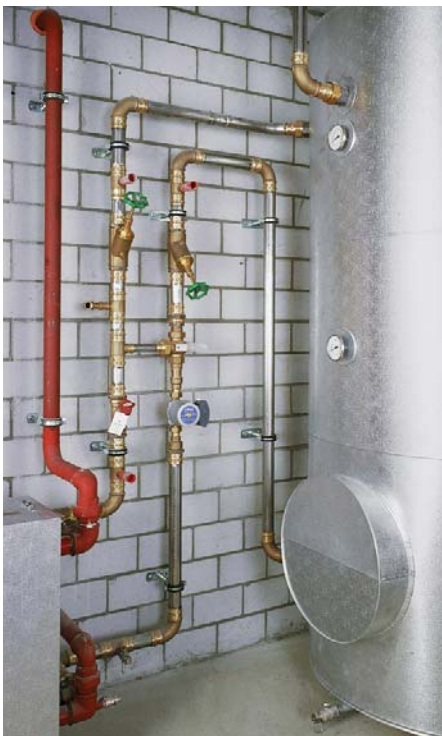
A professional hot water installation using Optipress.
