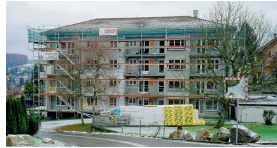
The almost 40-year-old block of flats undergoes complete renovation
